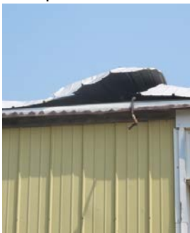
The roof that was damaged as the compressed air tank launched itself vertically.
