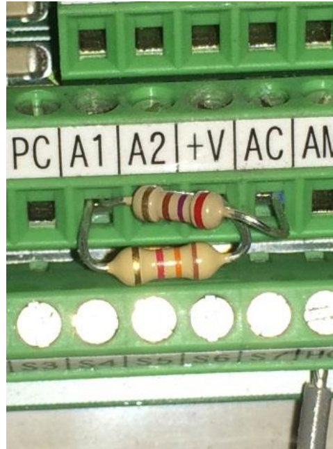
Figure A-9. Voltage divider resistors installed in the Yaskawa V1000 VFD terminals
