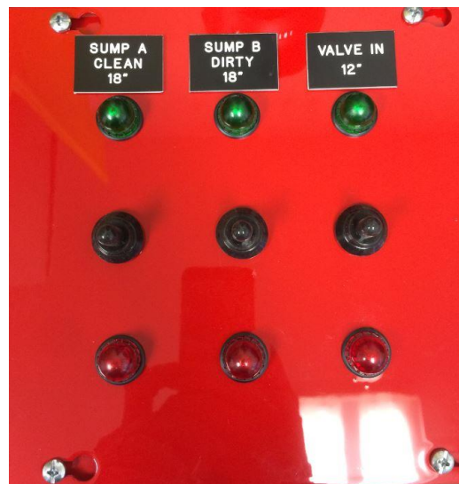
Figure A-5. Valve Control Toggle Switch Box
